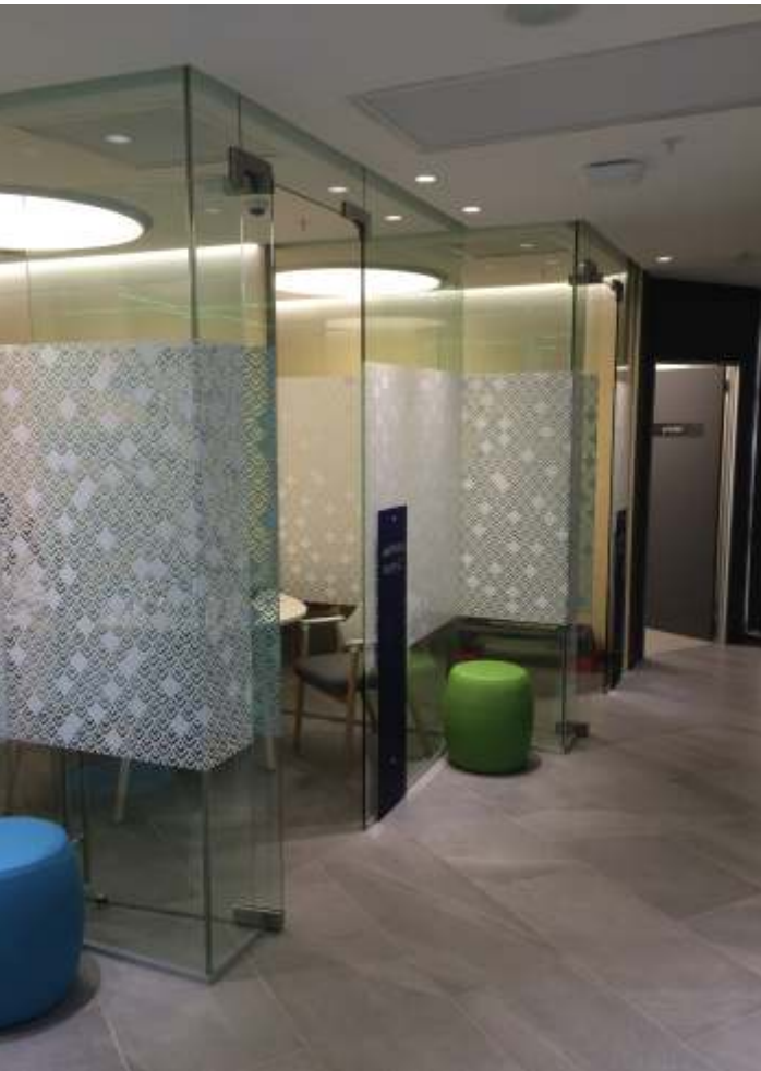
Left: Discovery Store, patch fitting doors with a glass toplight.
